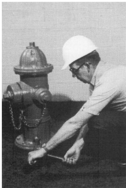
1. Loosen Nuts on Safety Flange Bolts.
