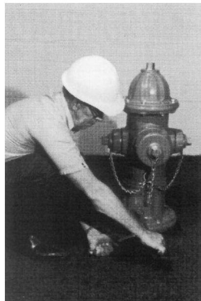
5. Tighten Safety Flange Bolts.
