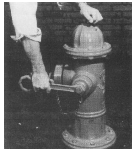
7. Replace and tighten Nozzle Cap.
