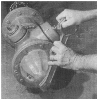
1. Tighten Operating Nut to be sure Main Valve is in the fully closed position.
