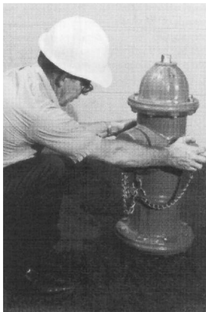
3. Rotate Upper Barrel section as desired.
